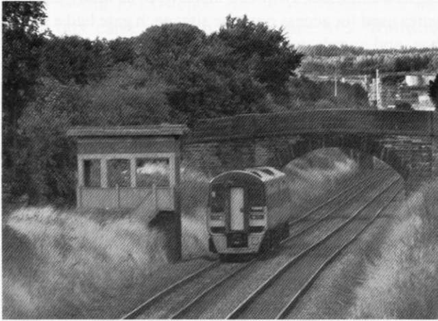
No. 2 ARP signal box.
